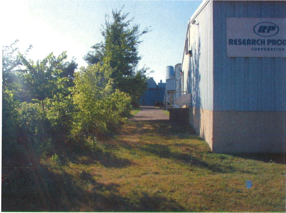
P1010009 Looking northwest toward E Main Street parcels from the southeast corner of 204 S Ingersoll Street. Showing the back of the Research Products buildings at 204 and 210 S Ingersoll Street adjacent to 215 S Brearly Street.
