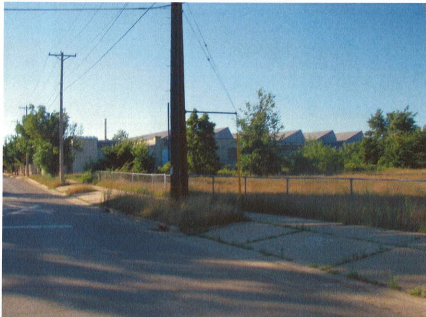
P1010002 Looking north at 211-255 S Brearly Street (former Byrns Property, a former petroleum bulk plant property) and the adjacent property to the north is 1011 E. Main Street, Research Products Corporation parcel and factory. A vacant parcel (255 S Brearly) separates the 211-215 S Brearly parcel from the 1011 E Main parcel and is near the tree line.
