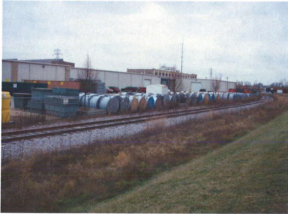
PC030009 Looking northwest from park property toward MG& E parcel and coiled cable and electric equipment storage on adjacent parcel to the north of the park.
