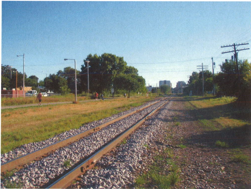
P1010010 Looking southwest toward S Brearly Street parcels from the railroad tracks adjacent to 204 S Ingersoll Street. Showing the adjacent parcel at 205 S Brearly Street and the adjacent bike/pedestrian path.
